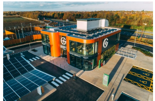
Figure 38: GRIDVOLT charging hub
